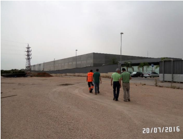
Indoor fresh solid waste treatment plant
